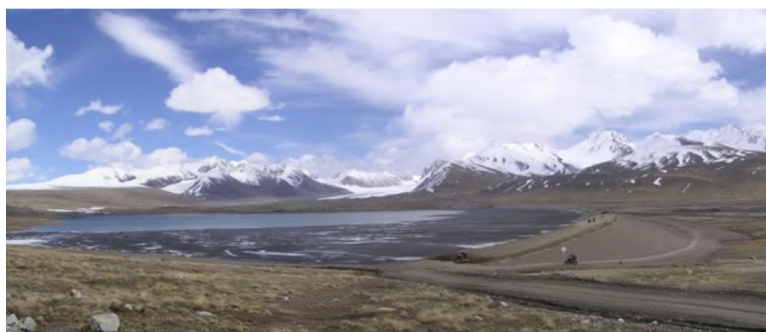
Figure 1. Kumtor tailings dam
